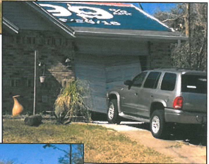
Garage door failure likely led to rapid pressurization of home (non-REBUILD home).
