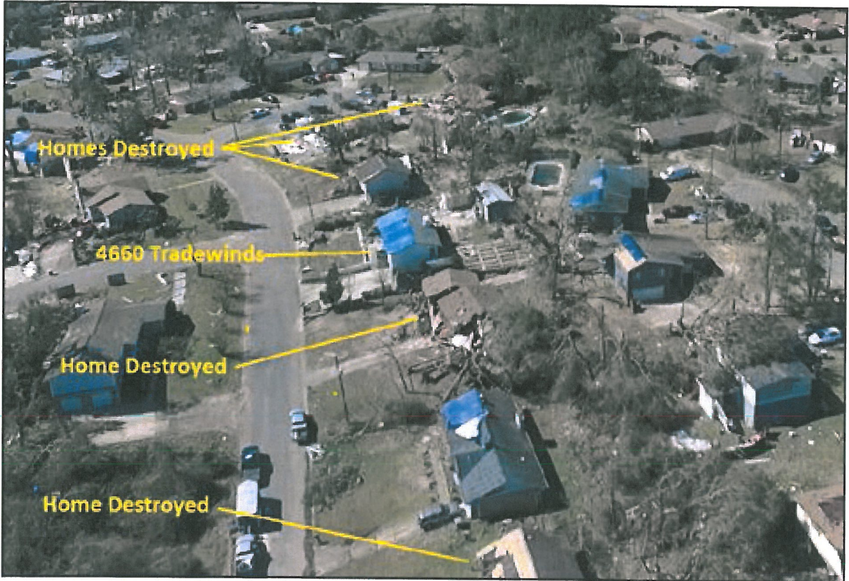
Drone view of 4660 Tradewinds Drive and surrounding non-REBUILD homes
