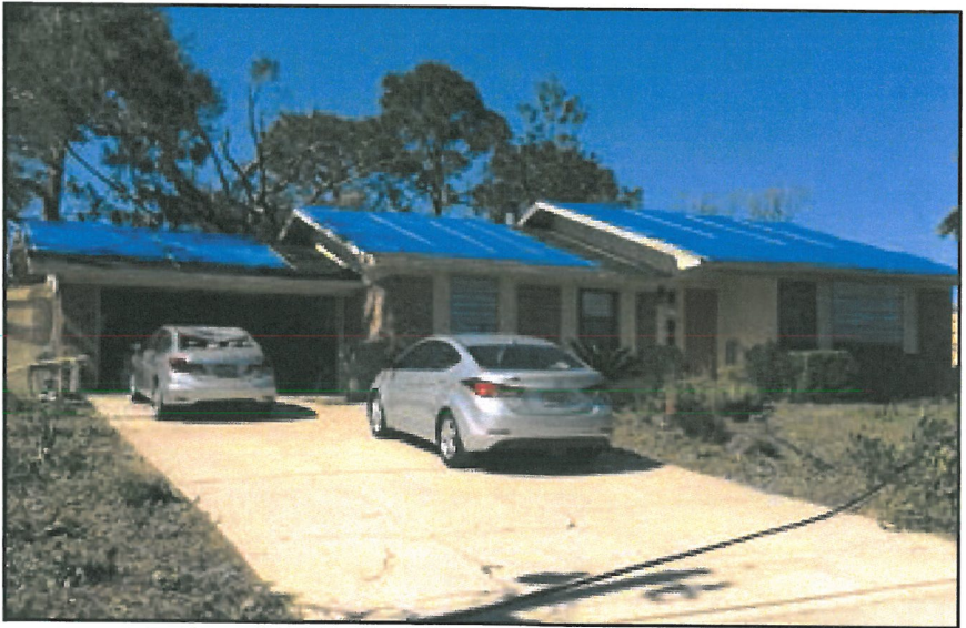
View of 4720 Tradewinds Drive after the tornado
