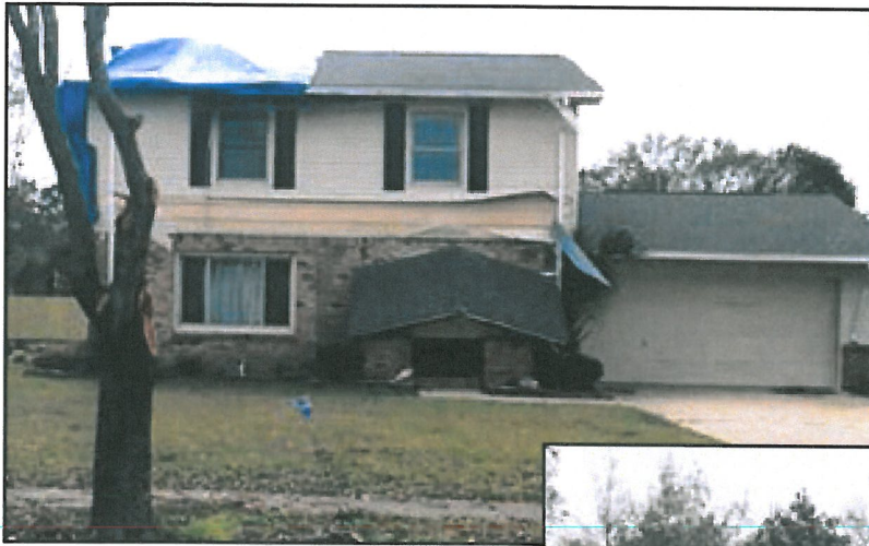
Heavily damaged/possibly destroyed homes across the street from 7800 Le Jeune Drive (non-REBUILD homes)
