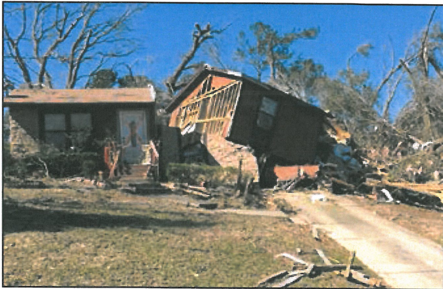
Destroyed home to the right of 4660 Tradewinds Drive (non-REBUILD home). The garage door's failure likely led to rapid pressurization of the home. We will discuss these and other failures in subsequent sections.
