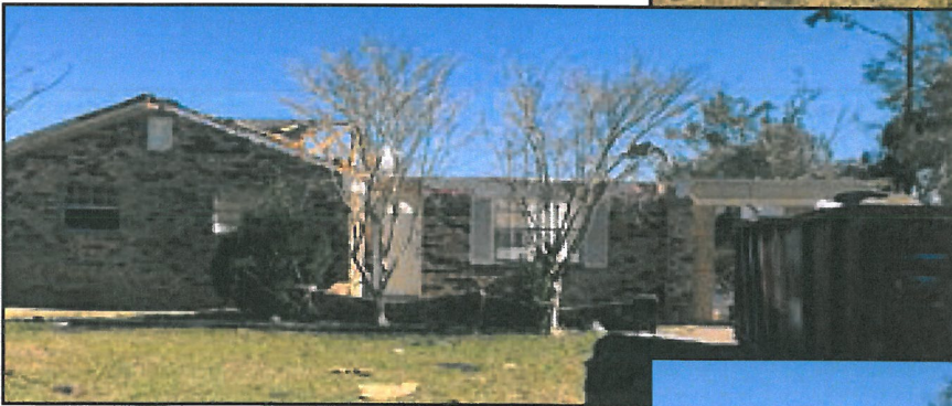
Garage door failure likely led to rapid pressurization of home (non-REBUILD home).
