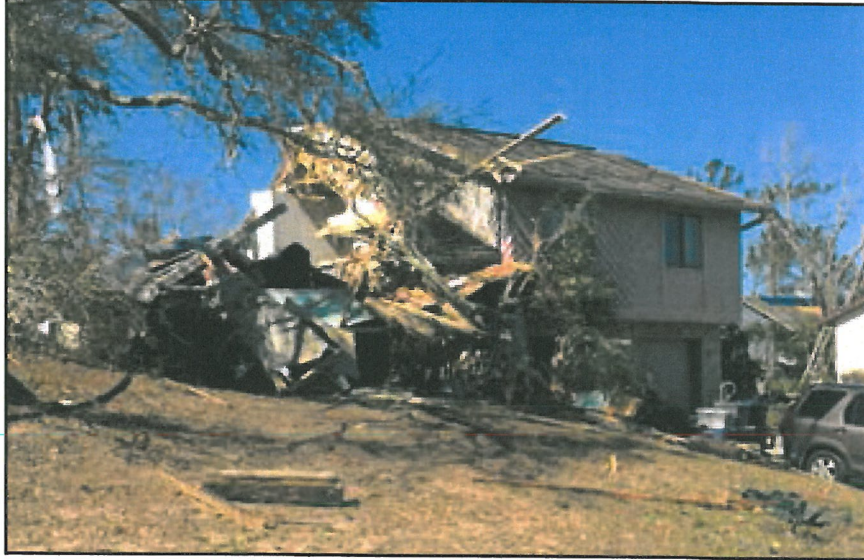
Destroyed home to the left of 4660 Tradewinds Drive (non-REBUILD home)
